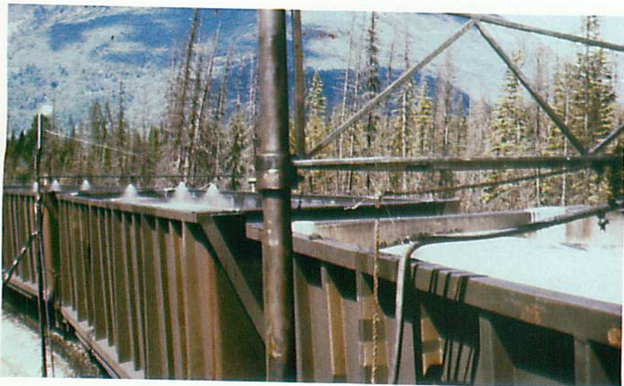
◀ PLATE NO.15: ADDITIONAL WATER SPRAYS TO INCREASE PENETRATION OF BINDER
