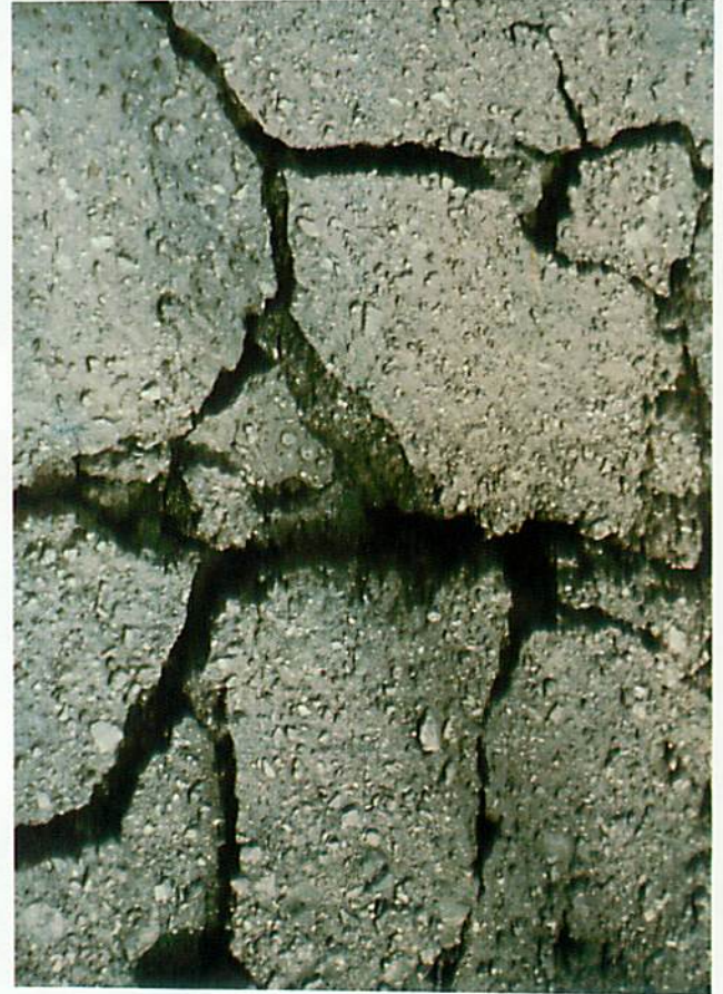
PLATE NO.11: CLOSE-UP SHOWING PENETRATION OF BINDER >
