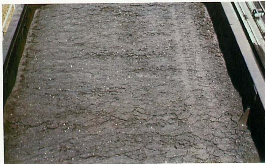
◀ PLATE NO. 18: PROPERLY LOADED AND SPRAYED SURFACE
