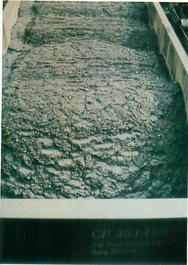
◀ PLATE NO. 19: EFFECTIVE SPRAYING ON AN UNEVEN PROFILE
