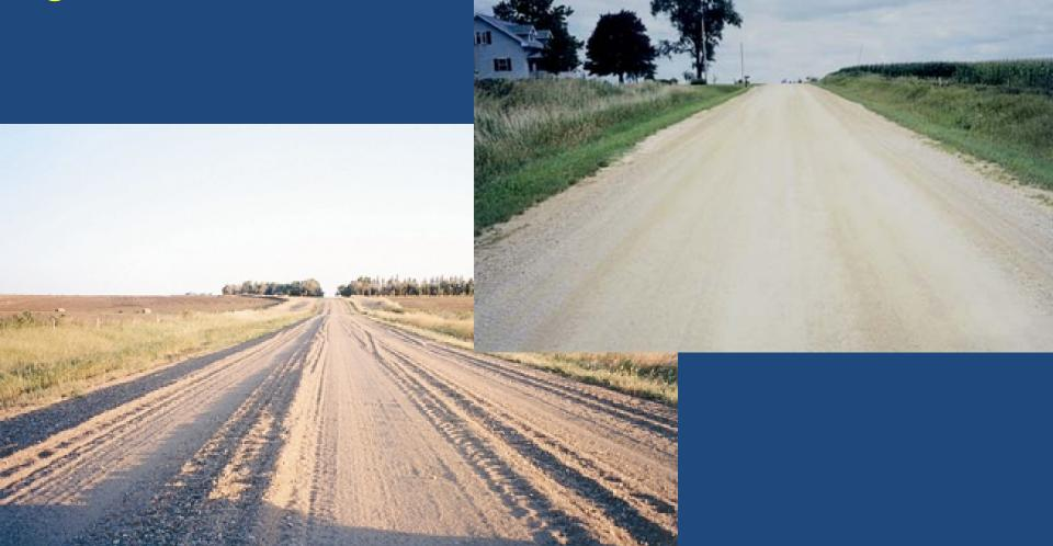
Dramatic difference in two surface aggregates in test done in Hand County, SD in 2002 & 2003
