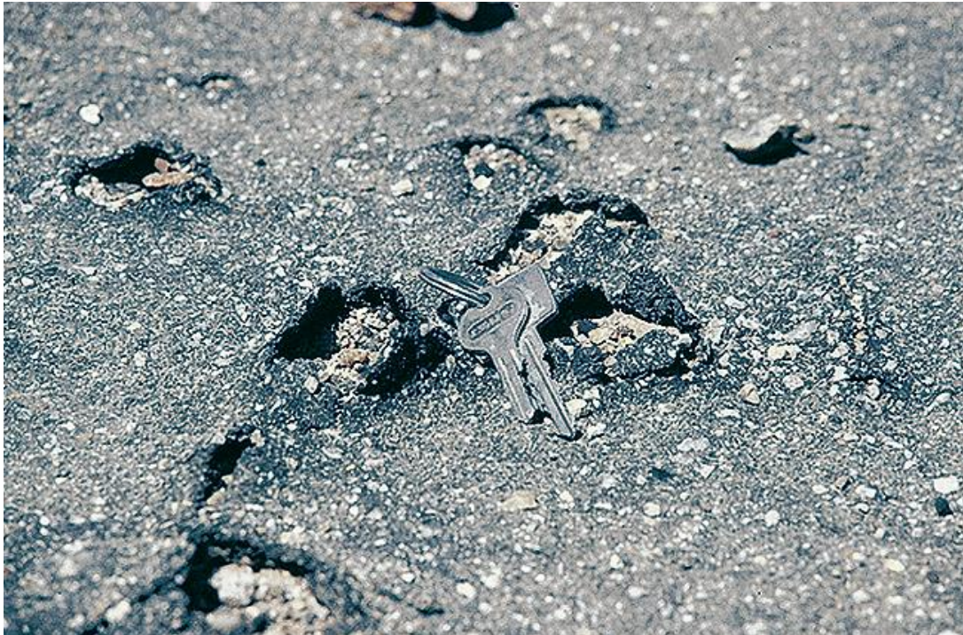
FIGURE 7: SALT BLISTER DAMAGE TO A PRIMED SURFACE IN BOTSWANA
